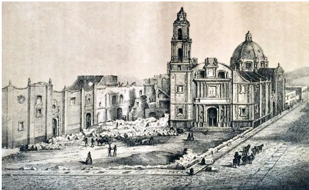
Figure 27: The partial demolition of the Santo Domingo cloister.
