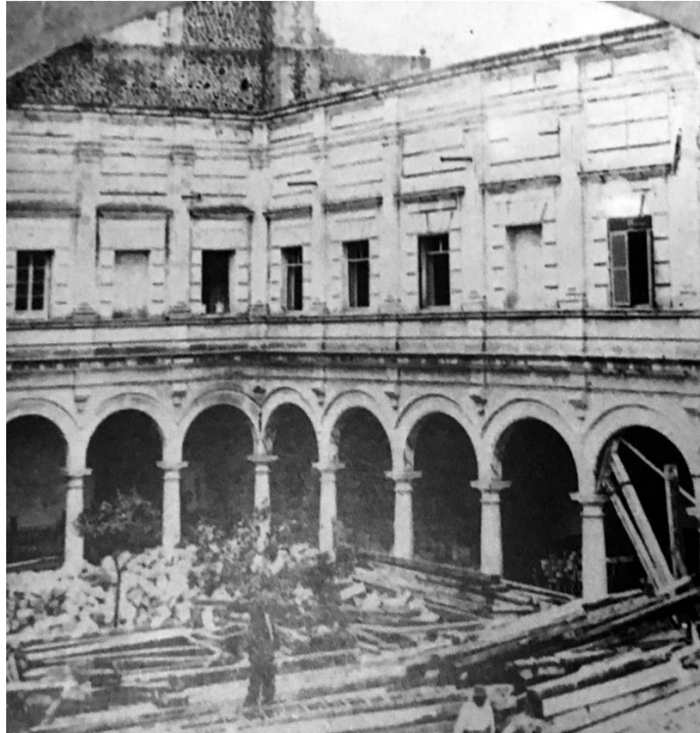
Figure 63: An 1861 photograph of the cloister of the casa profesa before its demolition.
