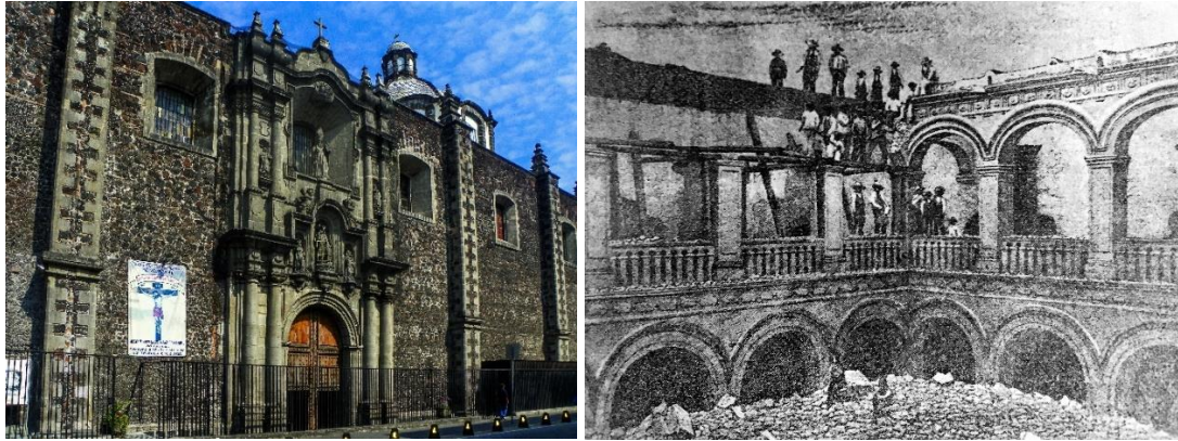
Figure 122: The San Lorenzo church and a historic photograph of the cloister before its demolition.
