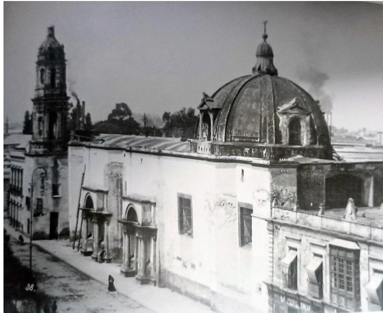
Figure 101: The Church of San Juan la Penitencia before its demolition.
