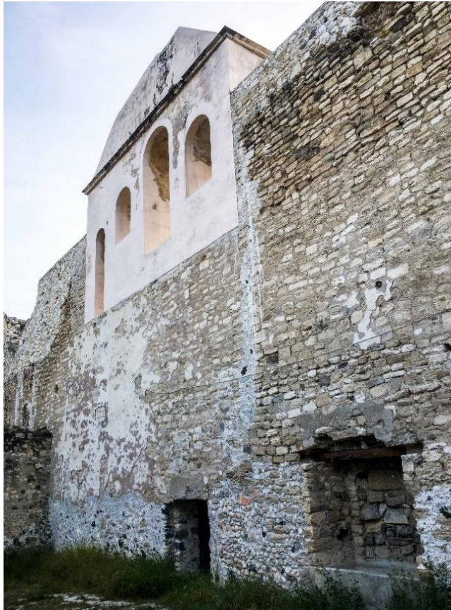
Figure 12: Detail of the church and espadaña showing the original roof line and new construction that raised the roof line when the church was reconstructed. Photograph in the collection of Robert H. Jackson.
