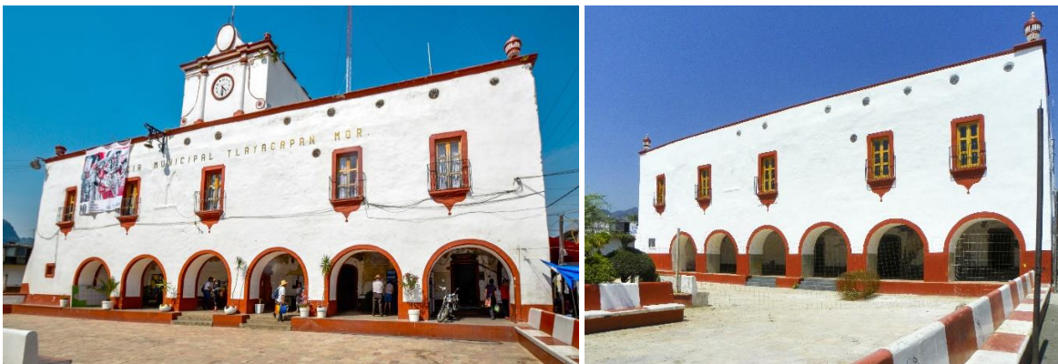
Figure 39: The Tlayacapan tecpán before the earthquake of September 19, 2017, and as reconstructed. Photographs in the collection of Robert H. Jackson.
