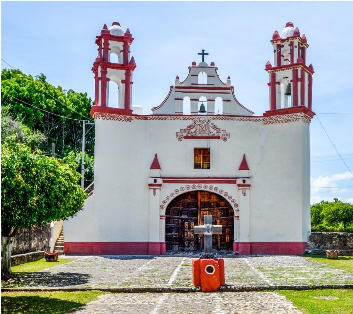
Figure 34: The barrio chapel dedicated to Sr. Santiago Apóstol that marks the eastern end of the east-west axis. The base of the atrial cross has a pre-Hispanic stone that depicts the sun. Photograph in the collection of Robert H. Jackson.
