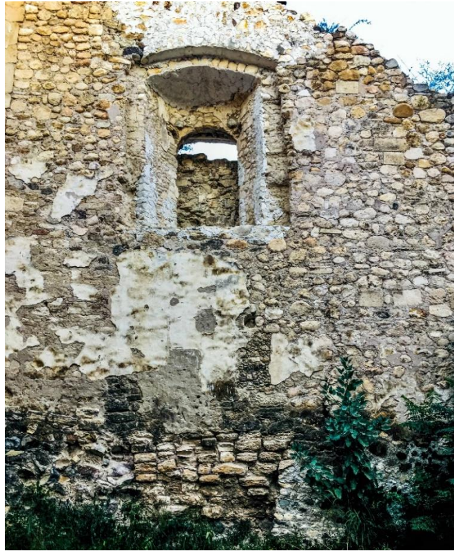
Figure 13: Detail showing the third arch that was later filled in when the “open chapel” was reconstructed and a window was added. Photograph in the collection of Robert H. Jackson.
