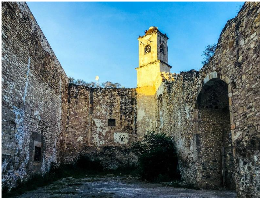
Figure 11: The nave of the church of La Comunidad, one entrance to the main square of the community, and the tower added in the mid-seventeenth century. It also shows the original roof line of the structure, and the later reconstruction that raised the roof line. Photograph in the collection of Robert H. Jackson.
