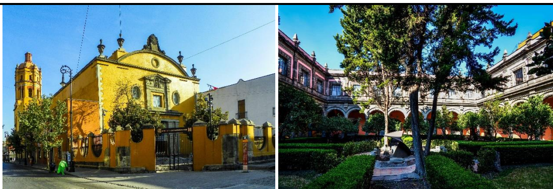
Figure 2: The church and main patio of the Colegio Máximo de San Pedro y San Pablo.
