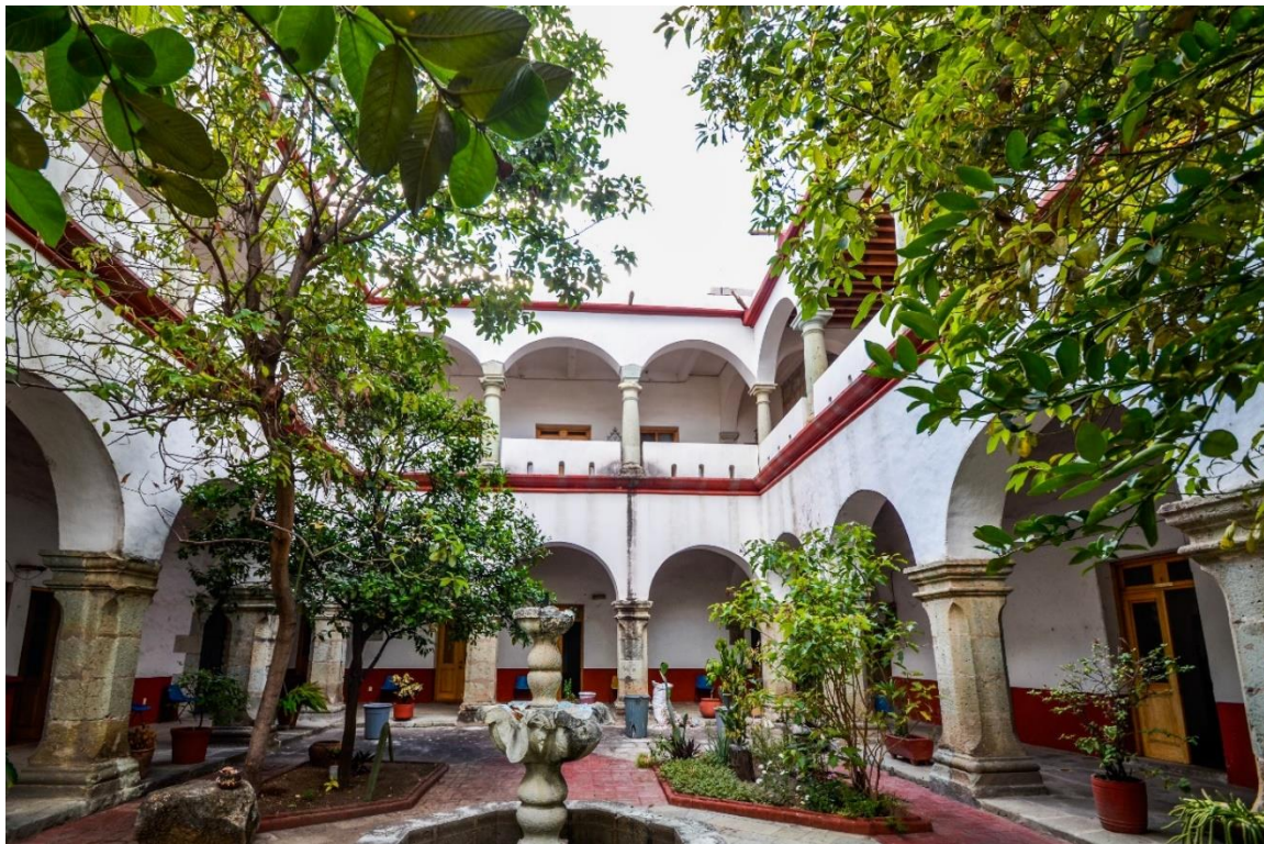
Figure 18: The first patio of the ex-colegio that serves as a parish office.
